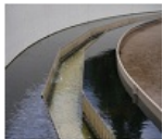
Fig. Sewage Treatment
