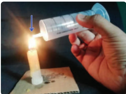
Fig. 7.12 , The syringe is heated and then pressed on a flat surface to close the tip of the syringe.
