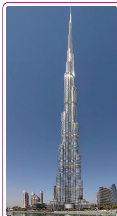
Fig. 2.1 , Burj Khalifa, an 828 m tall building located in Dubai; Image by King of Hearts via Wikipedia
