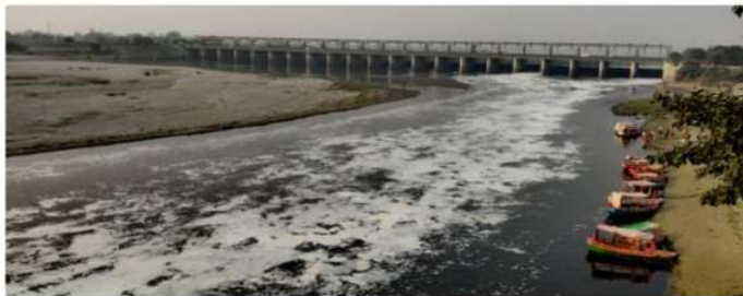
Industrial waste in river
