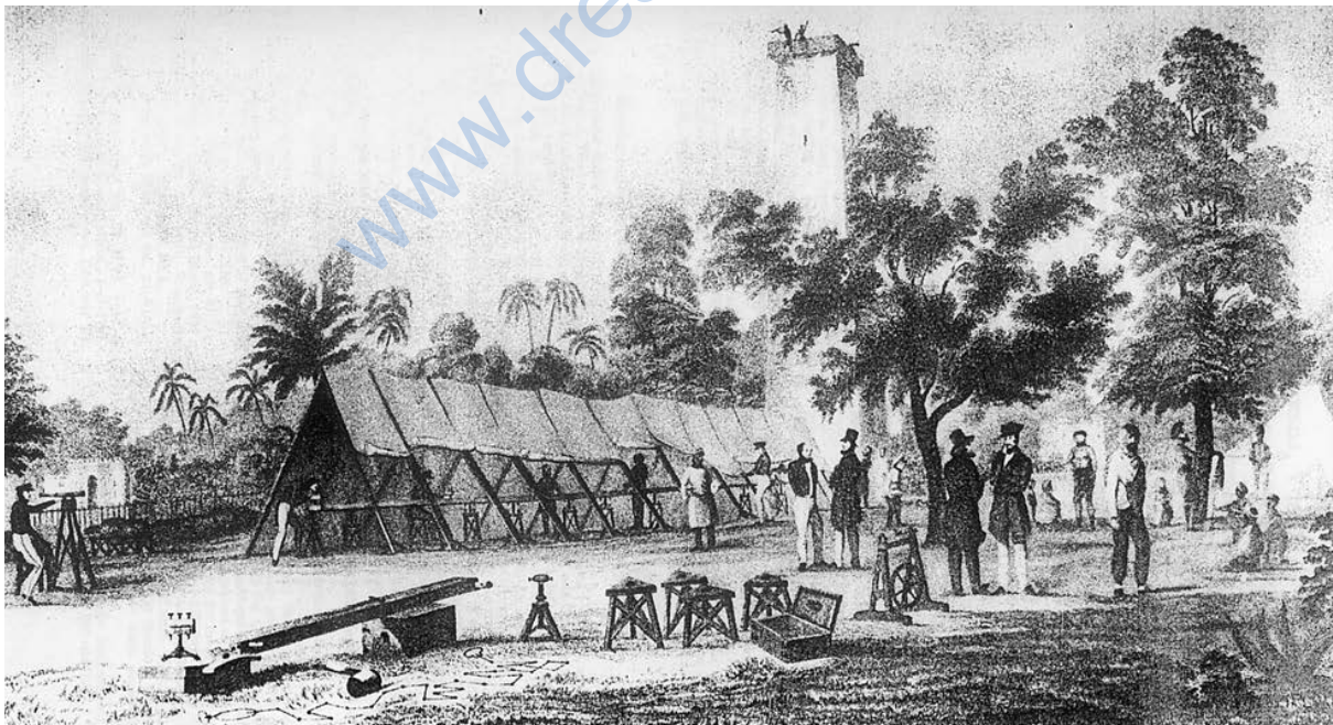
Fig. 6 – Mapping and survey operations in progress in Bengal, a drawing by James Prinsep, 1832
