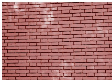
(a) Brick wall
